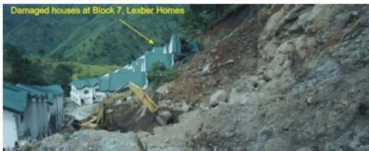
Increase in Total Construction Cost when Recommended Mitigating Measures are not Followed: A Case Study of a Subdivision on Sloping Ground (Source: Raza, 2003)
