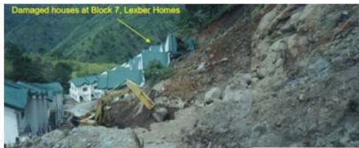
Increase in Total Construction Cost when Recommended Mitigating Measures are not Followed: A Case Study of a Subdivision on Sloping Ground (Source: Raza, 2003)
